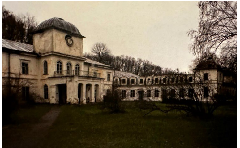
Figure 35 - Homutetz south facade 2012
