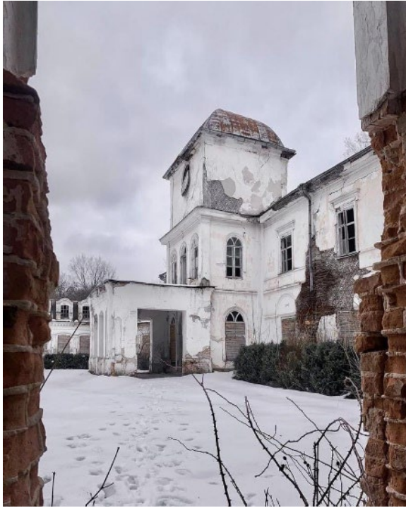
Figure 36 - Homutetz south facade 2020
