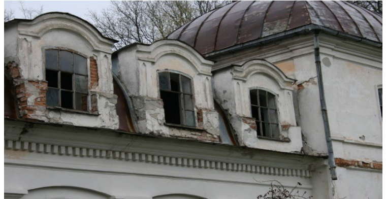
Figure 38 - Detail of 1820 addition construction
