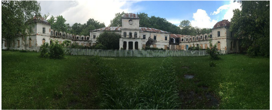
Figure 41 - Homutetz fenced off and boarded up after 2015
