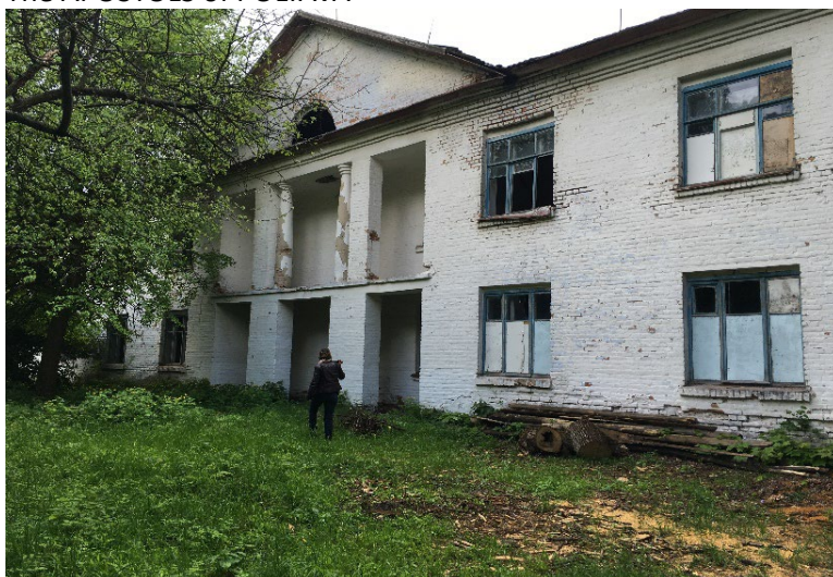
Figure 32 - Homutetz north facade 2018
