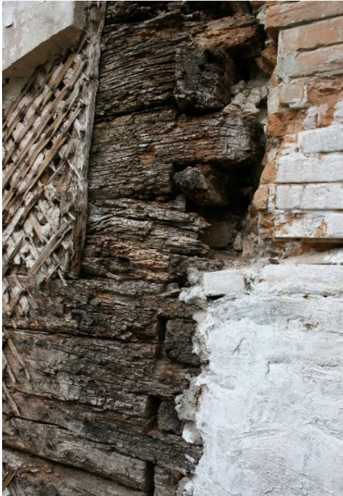
Figure 37 - Detail of original construction
