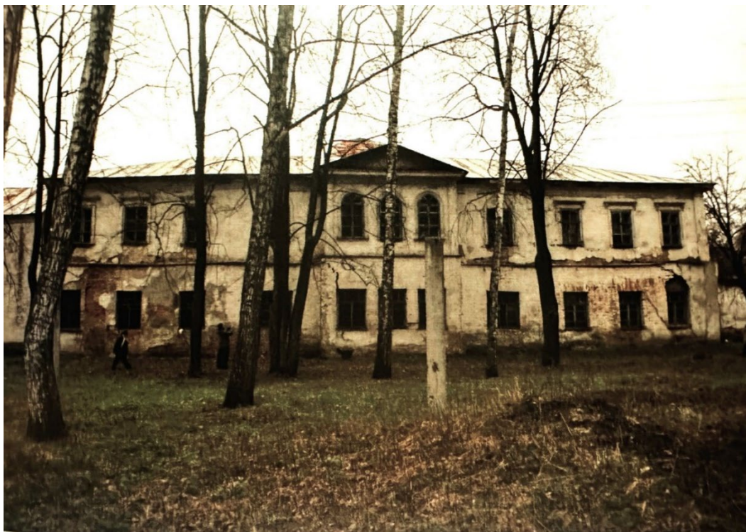
Figure 33 - Homutetz North facade 2012
